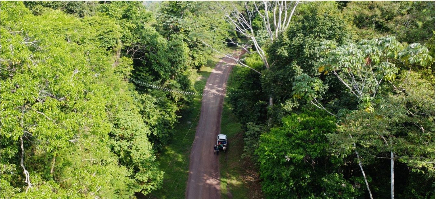
Aerial view of the Osa Peninsula landscape showing an installed arboreal bridge spanning an unpaved road. The bridge reconnects secondary forest patches on both sides of the road, providing a safe canopy-level crossing for arboreal mammals. Note the continuous forest cover extending beyond the road corridor—a key criterion for bridge site selection.
